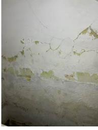
**Communal Areas:** Elevated damp readings and signs of water damage were recorded at low levels in the walls in the Entrance Hallways and stairwell. External defects to the bridged DPC and flooding to the basement below are almost certainly responsible for these readings.
